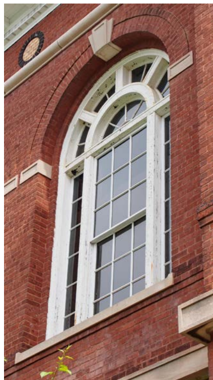
Second floor auditorium windows, double hung with fixed sidelights and fixed arch top. Paint is peeling.
