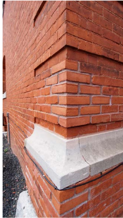
Example of brick repointing with inappropriate mortar. Such examples are rare.
