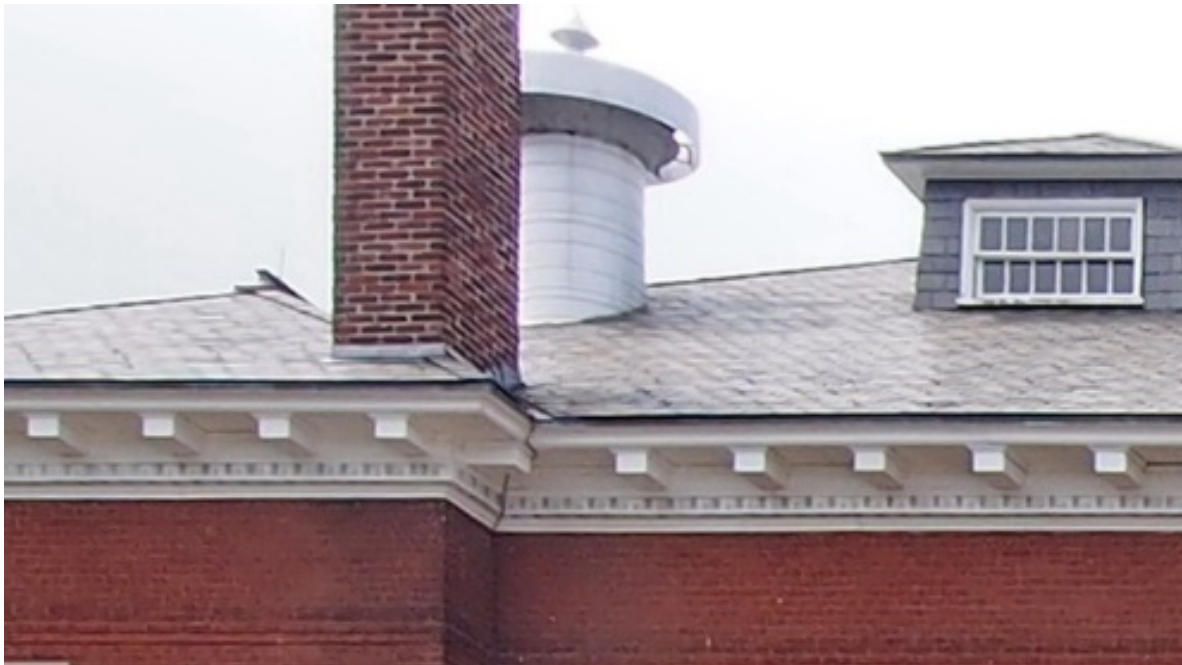
Slate roof showing penetrations. It is believed that slate that has loosened and fallen from the roof is slate that has been adhered, rather than nailed and was located at areas where slate meets the flashings at roof penetrations and dormer sidewalls.
