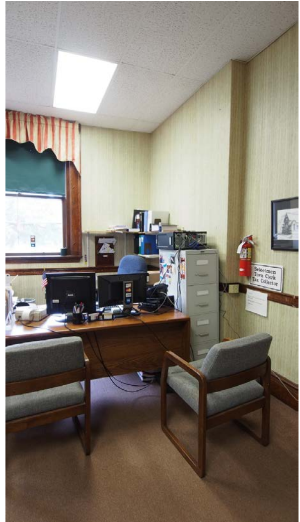
Typical office with carpet floor, textured wall paper, chairrail and hung ceiling tiles and fluorescent lighting.
