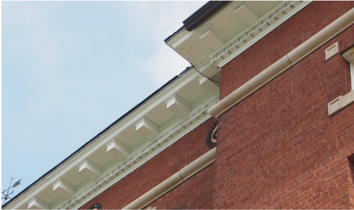
Painted soffit. Woodwork is in good condition, with paint holding up better than at windows.
