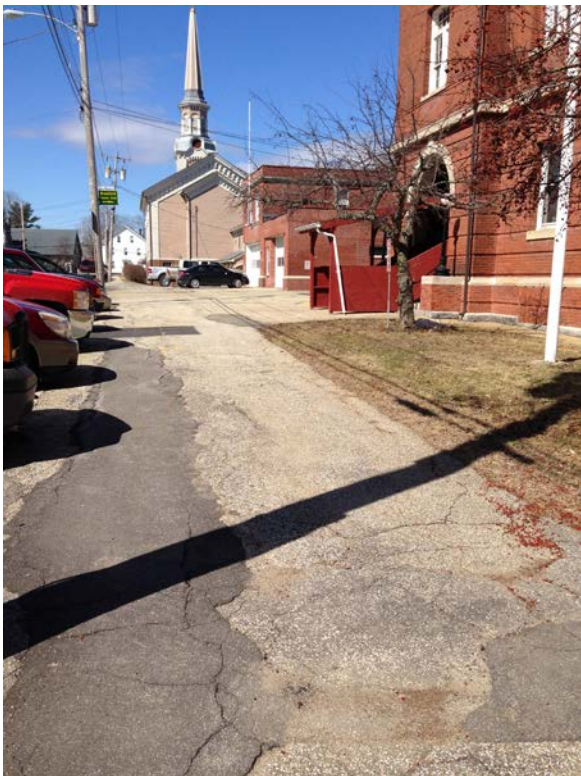
Walkways are deteriorated: Patched and uneven sidewalk at front of building.
