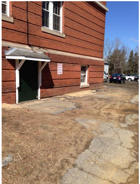
Walkways are deteriorated and dangerous: Asphalt paving and concrete walk at side service entrance.
