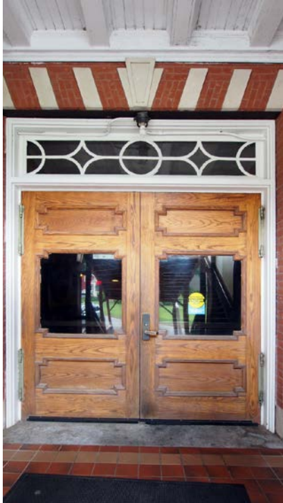
Front entry doors in recessed alcove. Masonry joints are tight, floor tile is in good conditions. Oak doors need to be refinished.
