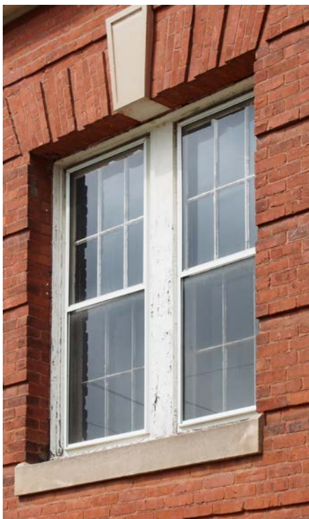
First floor windows in pedimented opening. Paint is peeling
