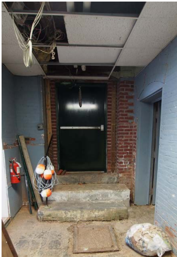
Basement hallway and egress/ service entry door. Note interior brick bearing walls. Stairs to exit intrude on egress to and from stairs to first floor on right.
