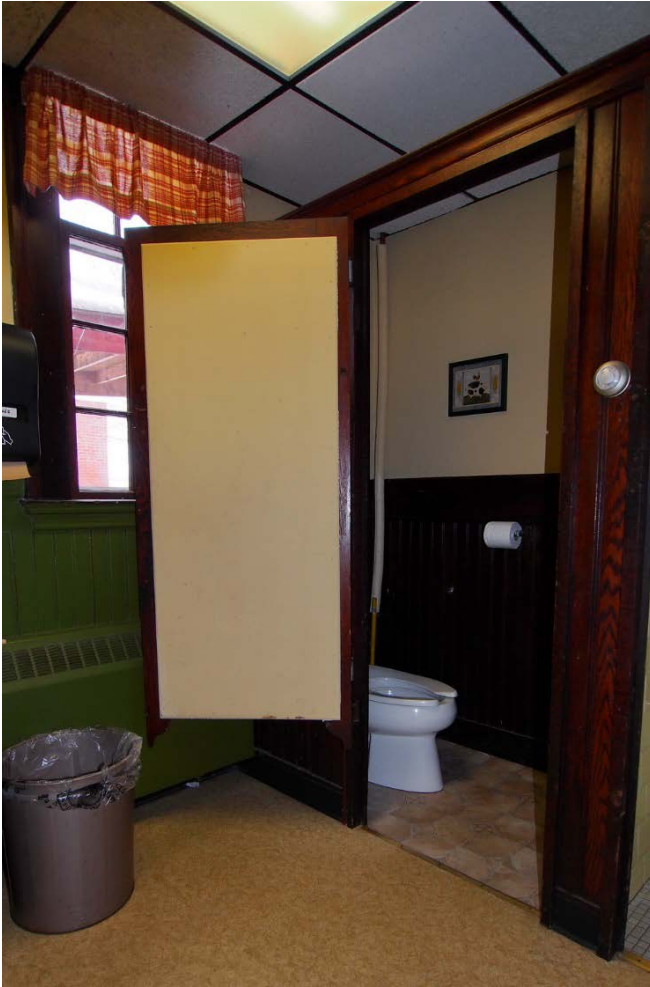
The sole toilet room on the first floor has one toilet stall and one urinal. Ceiling is hung tile, floor is sheet vinyl.
