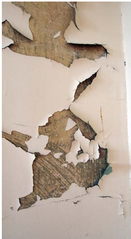
Peeling paint detail.
