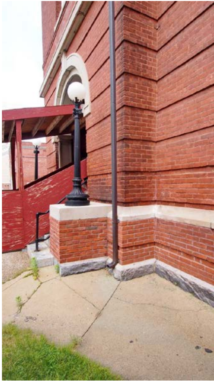
Detail of granite base, brick coursing and sandstone banding. Brick at lower levels has been repointed.
