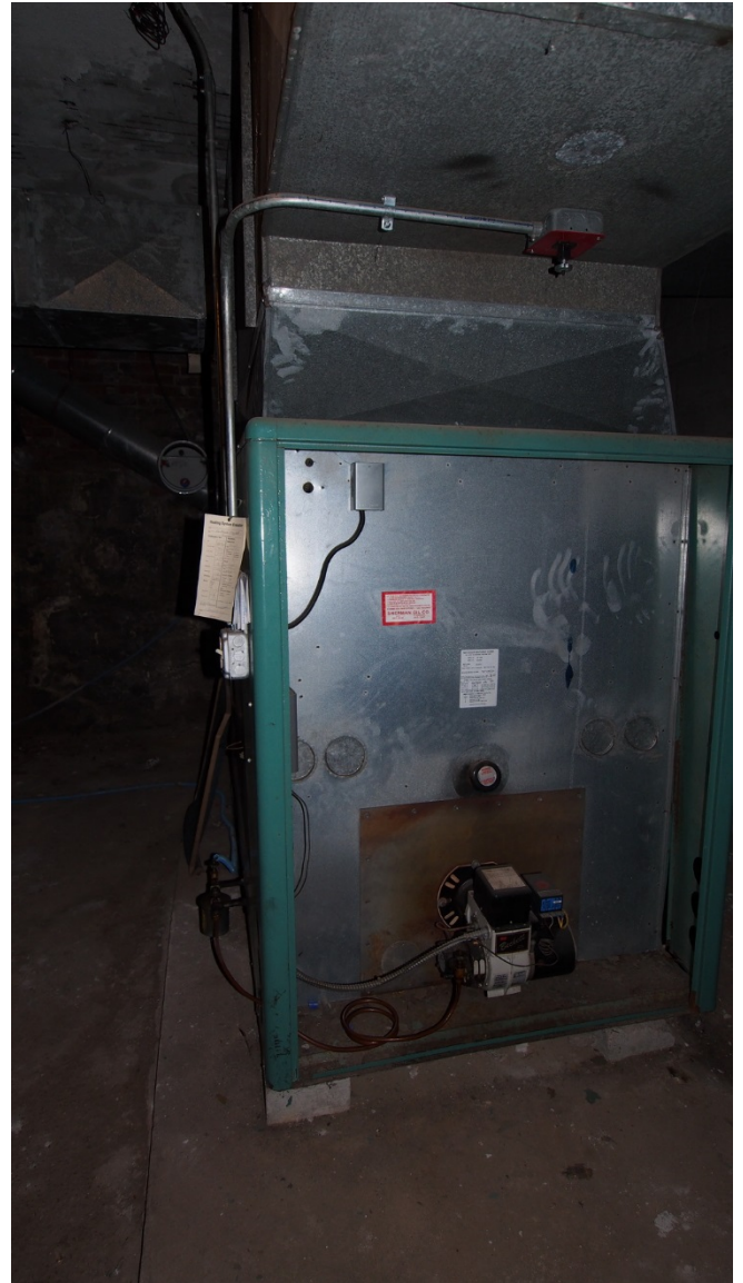
Furnace: Metzger Hot Air Furnace Model AFG (Purchased in 1999)
