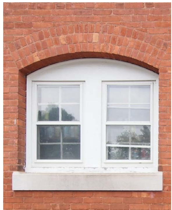
First floor windows with arched brick opening and sandstone sill. Storm windows have been applied over existing.
