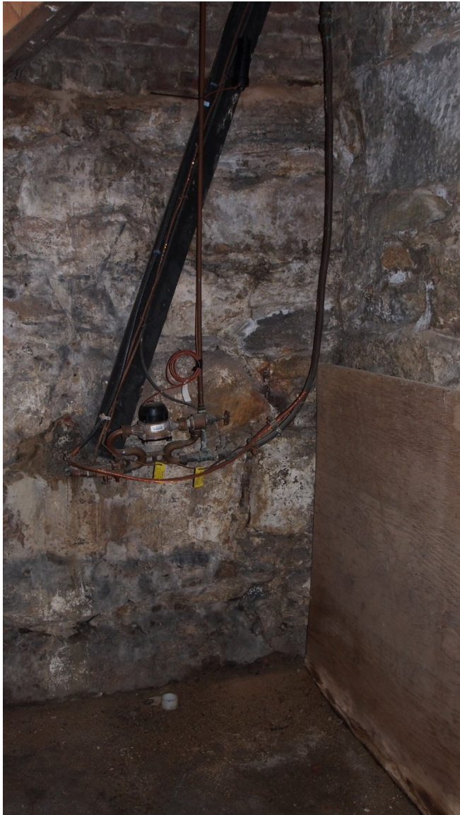
Water service entering on South west corner.
