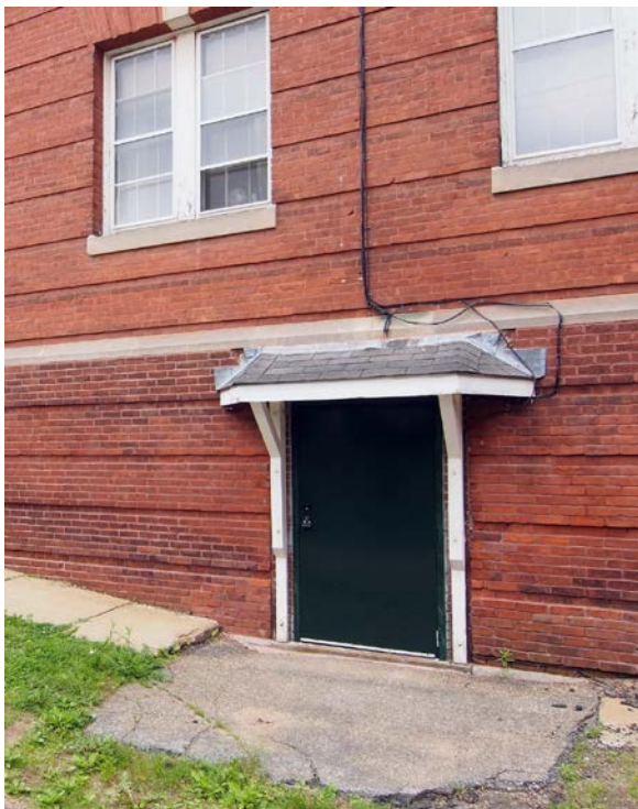
East end entrance to basement showing low doorway and deteriorated walkway
