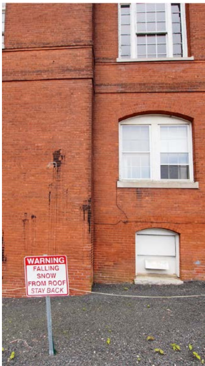
Masonry in need of cleaning, North façade.
