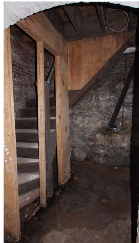
Stone foundation, brick knee wall and floor joists are visible. Former stairs that led to first floor, but are now closed off are located where new elevator is proposed to be installed. Signs of moisture are visible on the wall and floor.
