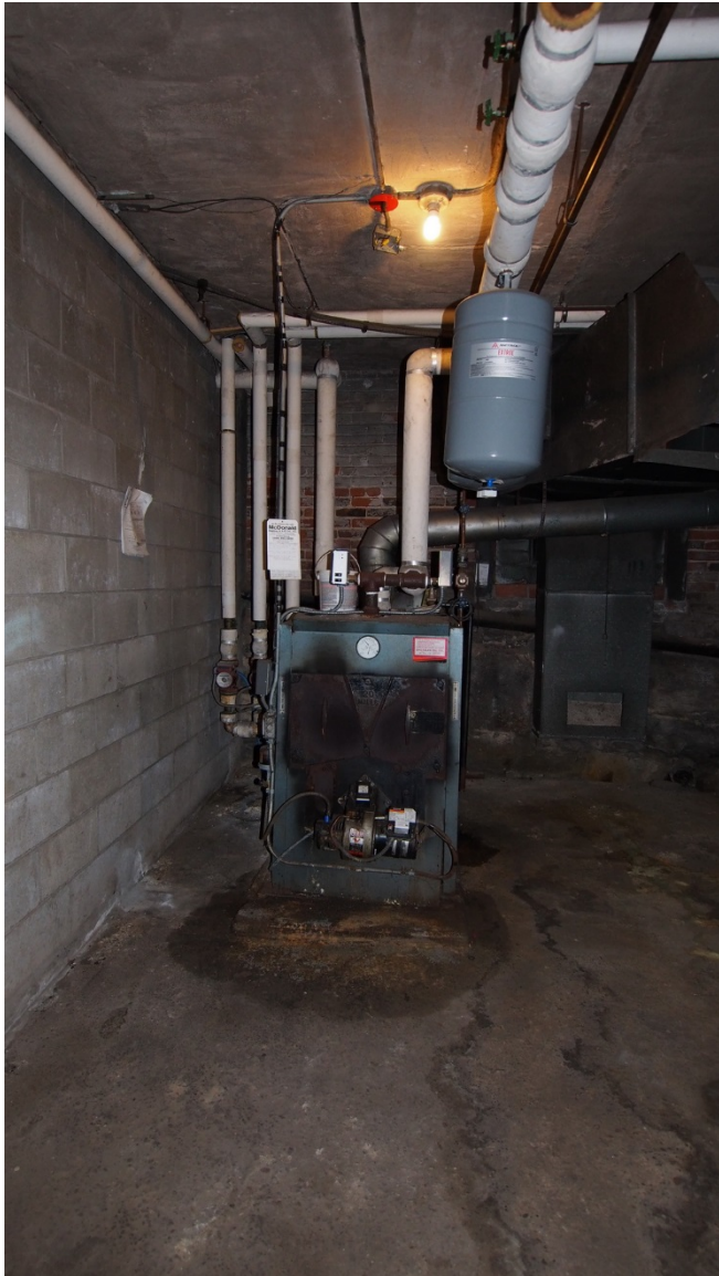
Boiler: Carlin Oil Burner Model 200CRD (Purchased in 1991)
