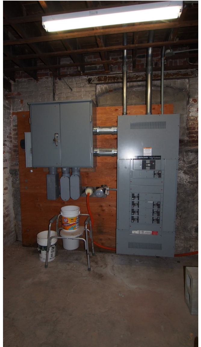
Electrical panels fed from underground service on South East corner.
