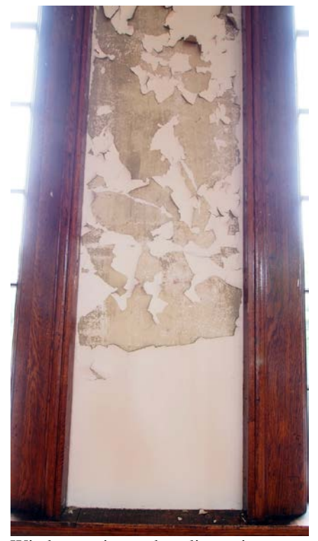
Window casing and peeling paint..
