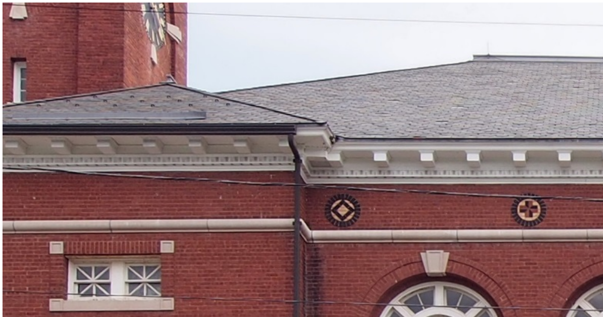
Slate roof showing snow deflector and guards over entrance. Additional, more effective snow guards and larger, copper gutter are recommended in lieu of the awning over the entrance below.
