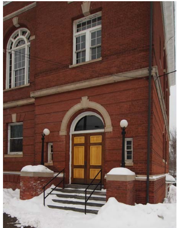
Secondary, front entrance. Doors swing out with no landing at top of stairs.
