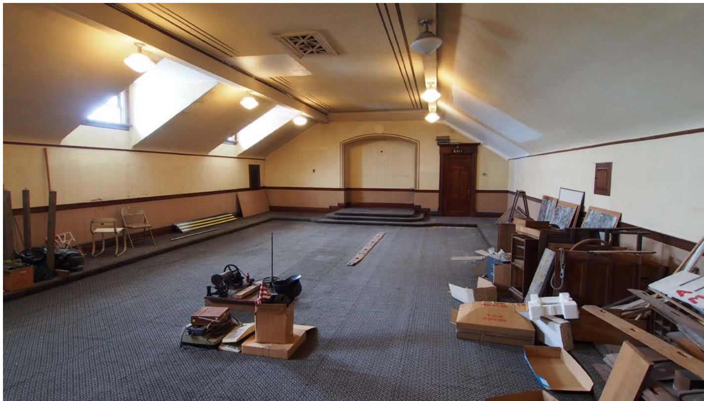
Main third floor space showing dormers and sloped rafter / ceiling plane.
