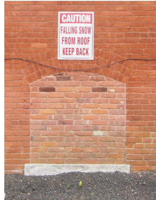
Window opening showing original arched brick lintel and brick infill.
