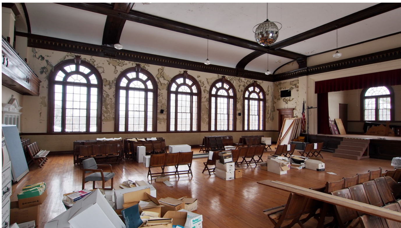
Main Auditorium space showing clear span of third floor – ceiling trusses.
