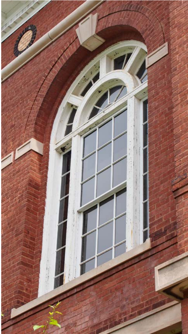
Arched brick opening at Second Floor Window
