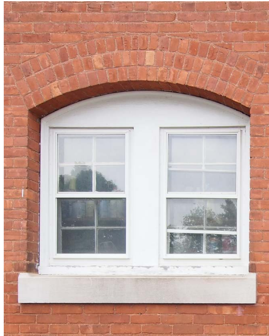
Arched brick opening at First Floor Window
