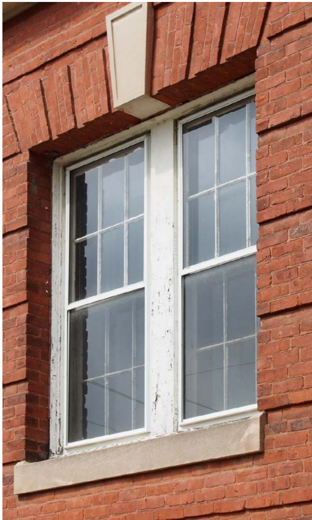
Pedimented brick opening at First Floor Window
