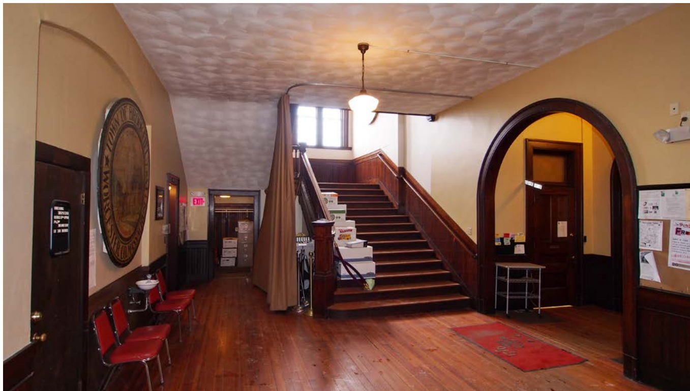
Main stair Hall with masonry partitions on side walls
