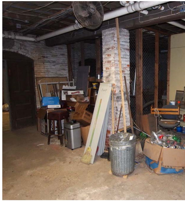
Arched opening, brick pier, wood beam and wood joists.
