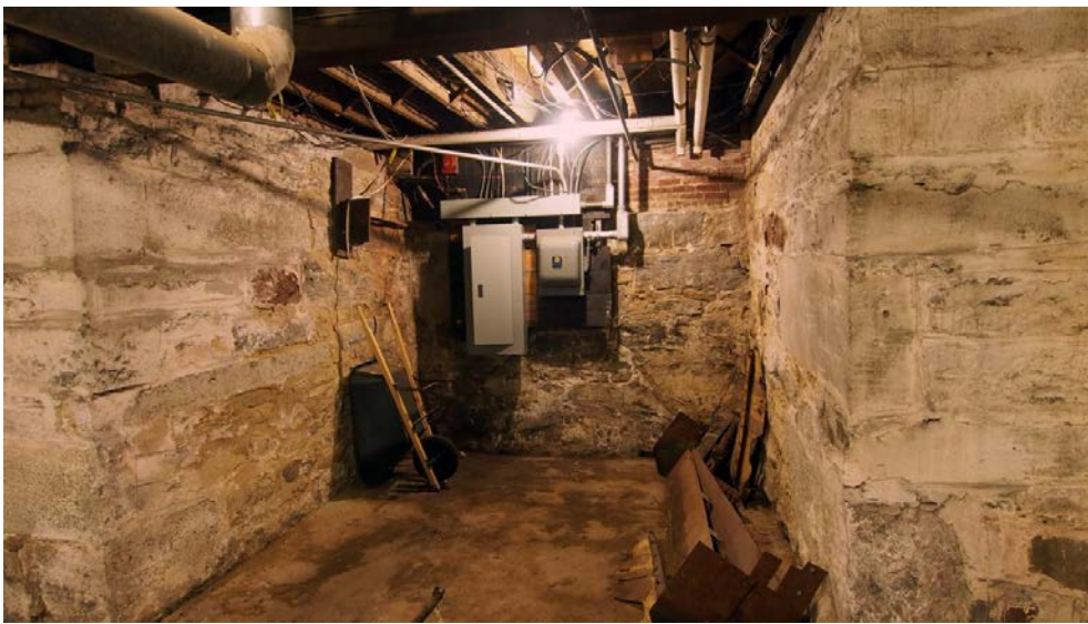
Stone foundation wall, brick knee wall above, 2x12 exposed floor joists
